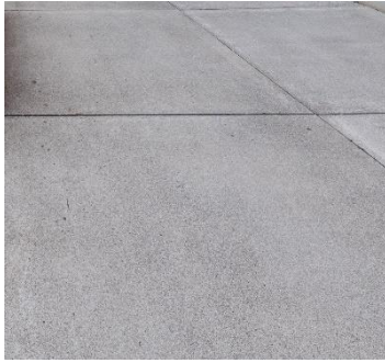
Plate 4-13 Example of concrete pavers/hardstanding
