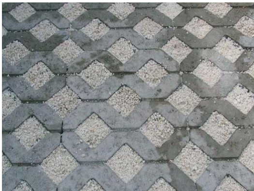
Plate 4-32 Example of filter drains and permeable surfaces
