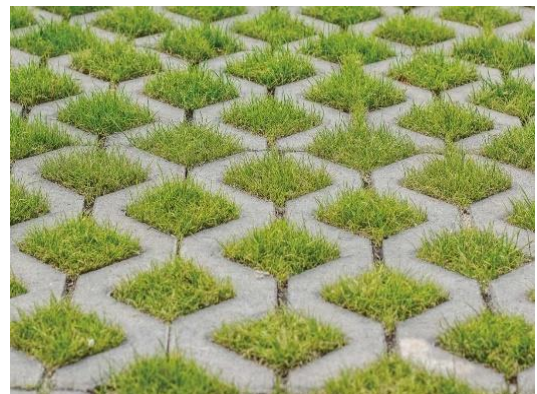
Plate 4-32 Example of filter drains and permeable surfaces
